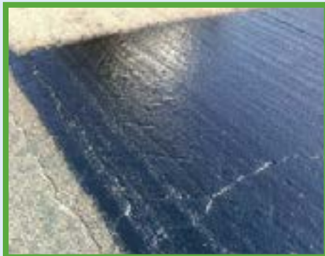
Properly applied tack coat
